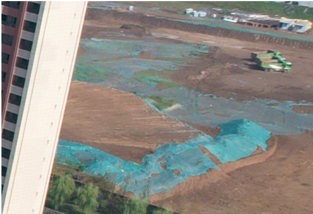
堆土临时苫盖
